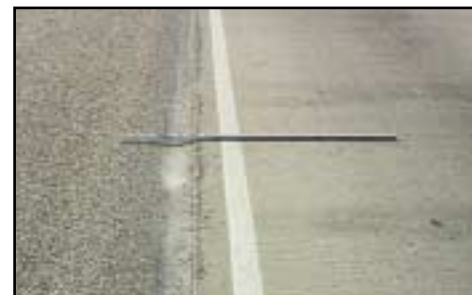
FIGURE 115 Distress Type CRCP 9—Lane-to-Shoulder Dropoff
