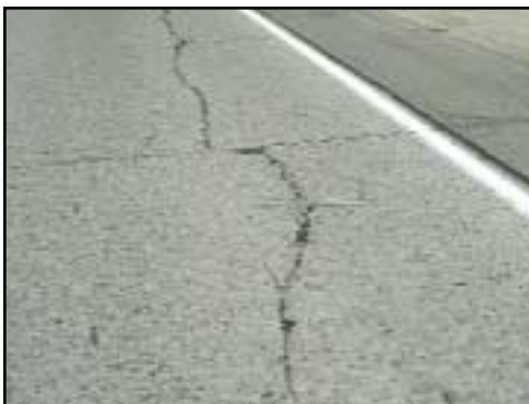
FIGURE 57 Distress Type JCP 3—High Severity Longitudinal Cracking
