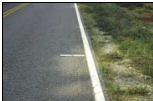
FIGURE 12 Distress Type ACP 3—Low Severity Edge Cracking
