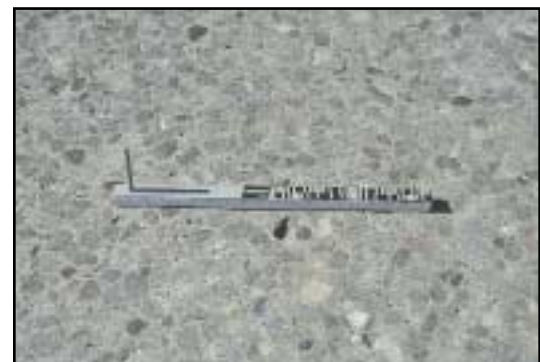
FIGURE 74 Distress Type JCP 10—A Popout
