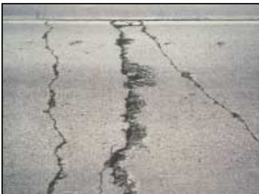
FIGURE 100 Distress Type CRCP 3—High Severity Transverse Cracking
