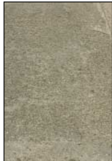
FIGURE 102 Distress Type CRCP 4b—Scaling
