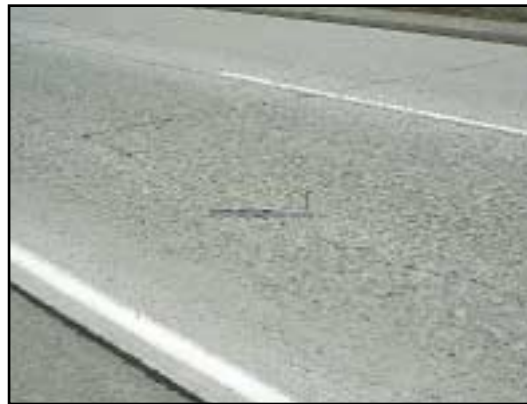
FIGURE 56 Distress Type JCP 3—Moderate Severity Longitudinal Cracking
