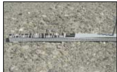
FIGURE 42 Distress Type ACP 13—Loss of Coarse Aggregate
