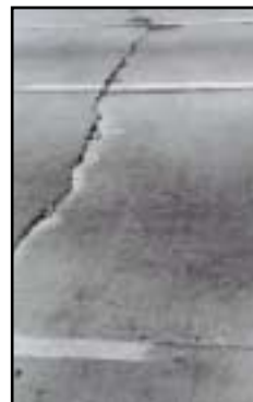
FIGURE 78 Distress Type JCP 12—Faulting of Transverse Cracks
